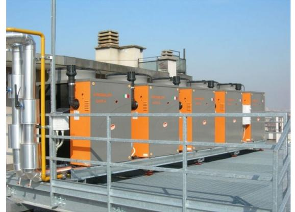
electric strip heaters/humidifiers. Many bakeries have been searching for alternatives to steam boilers due to maintenance requirements and boiler chemical use in a food processing facility.
