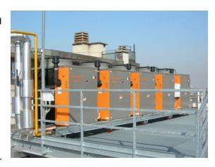
electric strip heaters/humidifiers. Many bakeries have been searching for alternatives to steam boilers due to maintenance requirements and boiler chemical use in a food processing facility.
